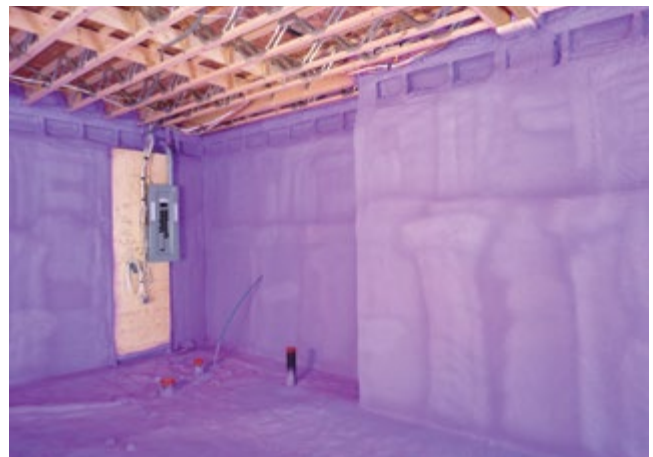
WALLTITE® CM01 applied on basement walls and under slab
