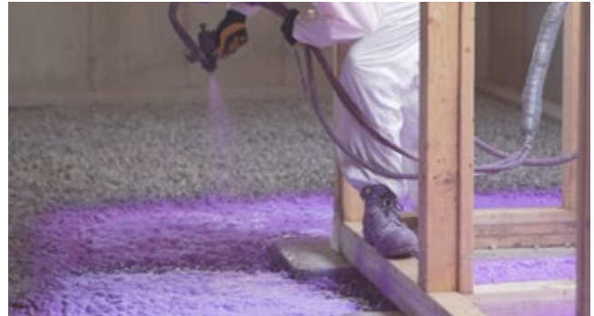
WALLTITE® CM01 sprayed directly on gravel for under slab
