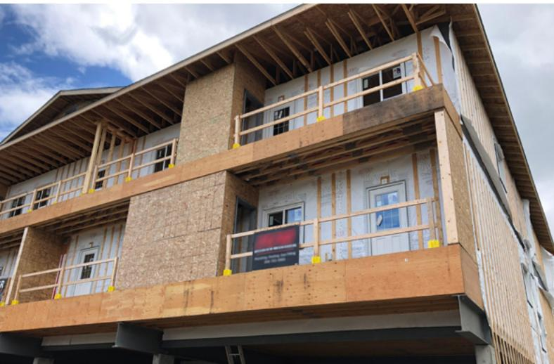
eliminating thermal bridging. Inside the wall cavity, WALLTITE was sprayed to provide additional insulation and to be the air/vapour barrier. What was the result? For this XR wall system, an RSI of 5.45 (R-value 30.9) was achieved. While based on typical 2 x 4' wood framing, there are some differences between standard building practices and assembling an XR wall; differences that improve the overall building envelope.
