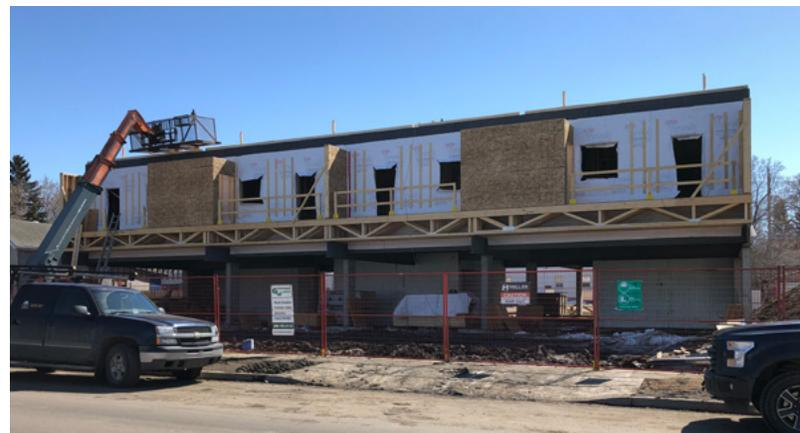
Attached to the exterior of the framing, Neopor sheets were fastened to provide continuous insulation;
