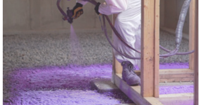
WALLTITE® sprayed directly on gravel for under slab
